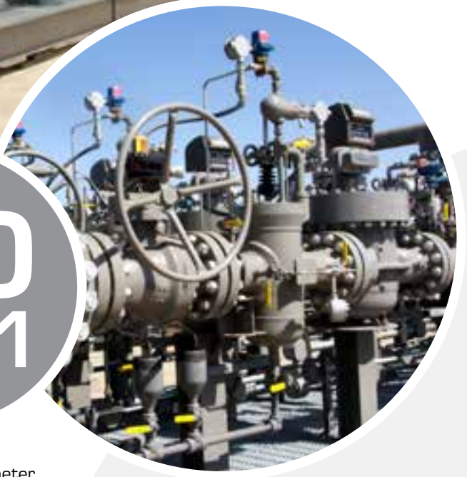
90 MMSCF/Day Gate station with scrubber, coalescer, gas meter skid, pressure reduction, heater, and control panel.
